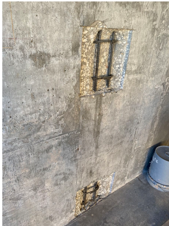
Picture 2: Typical divider wall repairs
