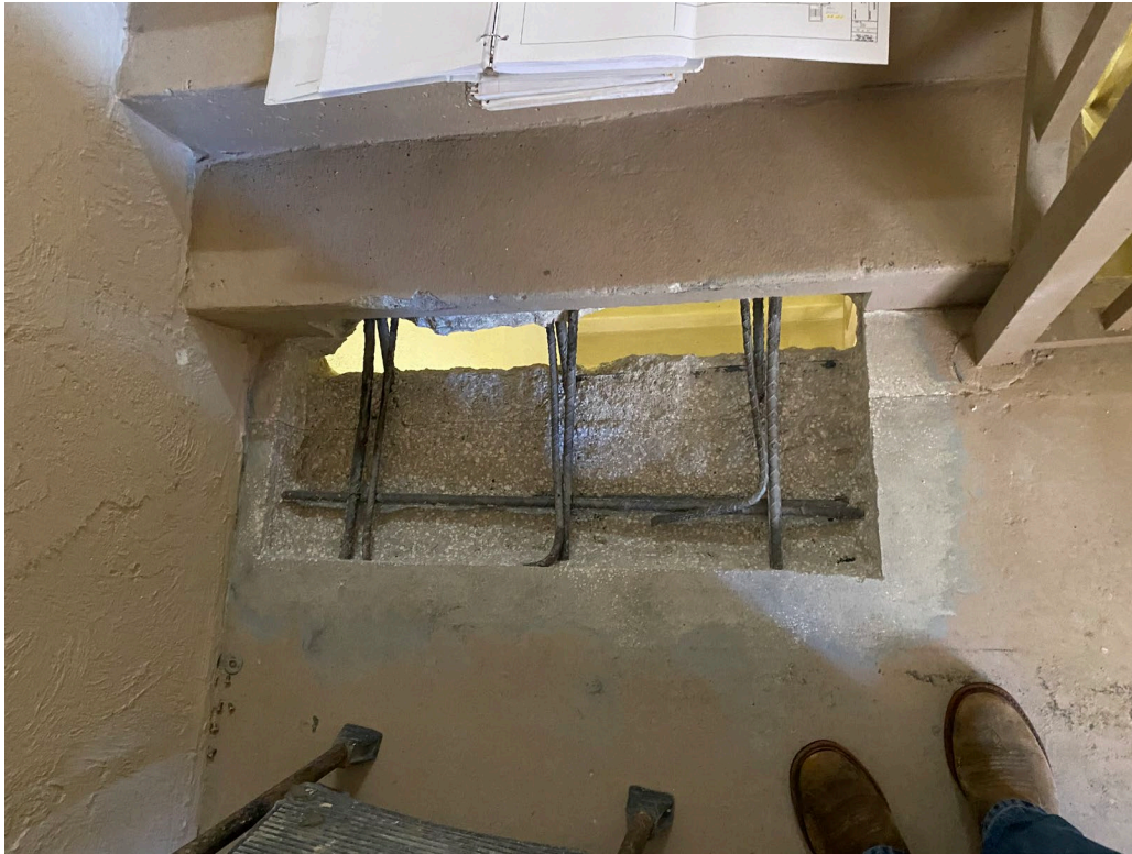
Picture 1: Repair in N. stairwell at the 7 th floor
