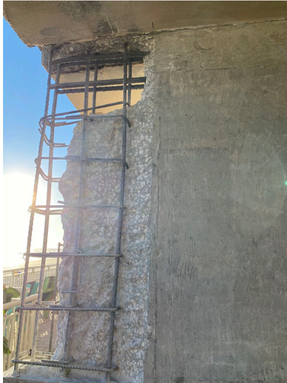
Picture 3: Typical divider end wall repair
